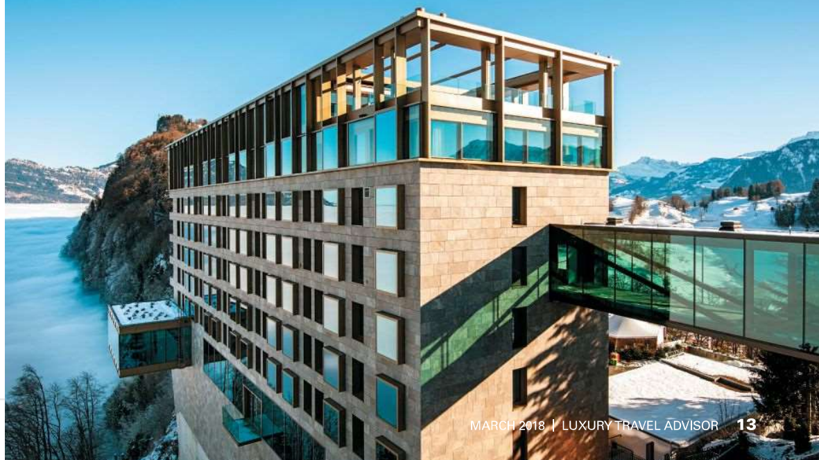
THE BÜRGENSTOCK HOTEL houses 102 rooms and suites with a view of Lake Lucerne.
